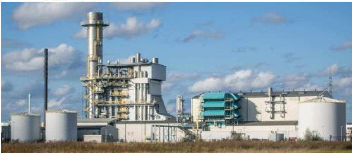
Figure 6: Photo of the gas power plant in Tessenderlo [10]
