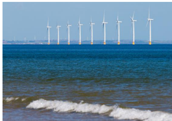
Figuur 10: off-shore windpark [19]
